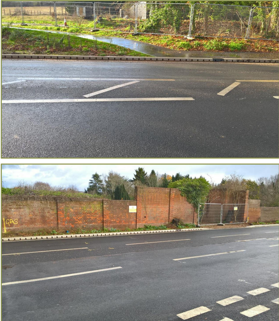
Beany blocks along eastern (top) and western (bottom) side of highway.
