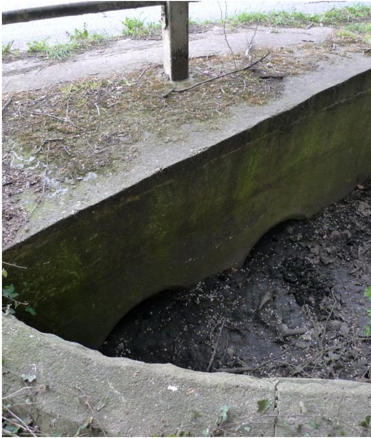
5. Downstream side of culvert under A4155
