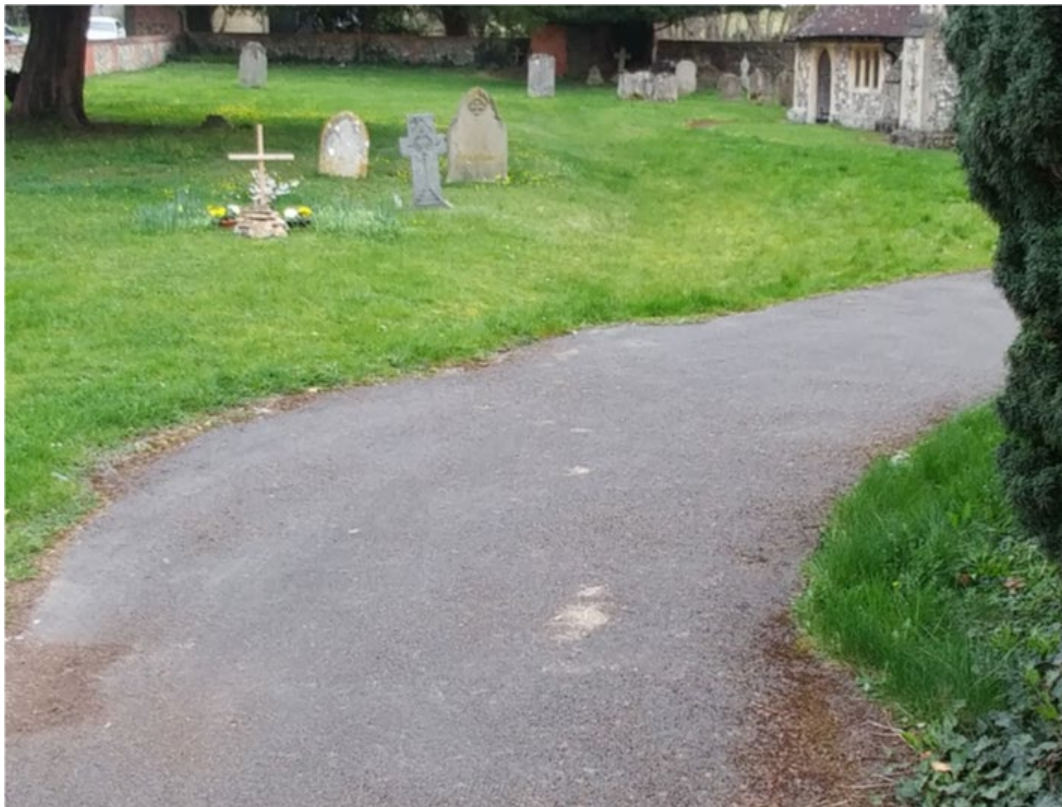
33. Path and drainage depression? Into churchyard just above Harpsden Court.
