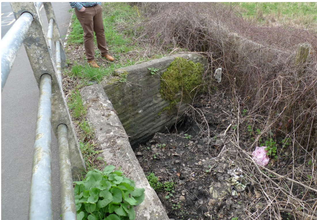
4. Upstream side of culvert under A4155 with road drain coming in from the south. (guess)
