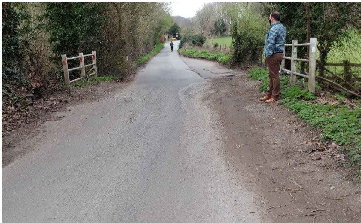
30. Road above culverted stream route. Regularly floods
