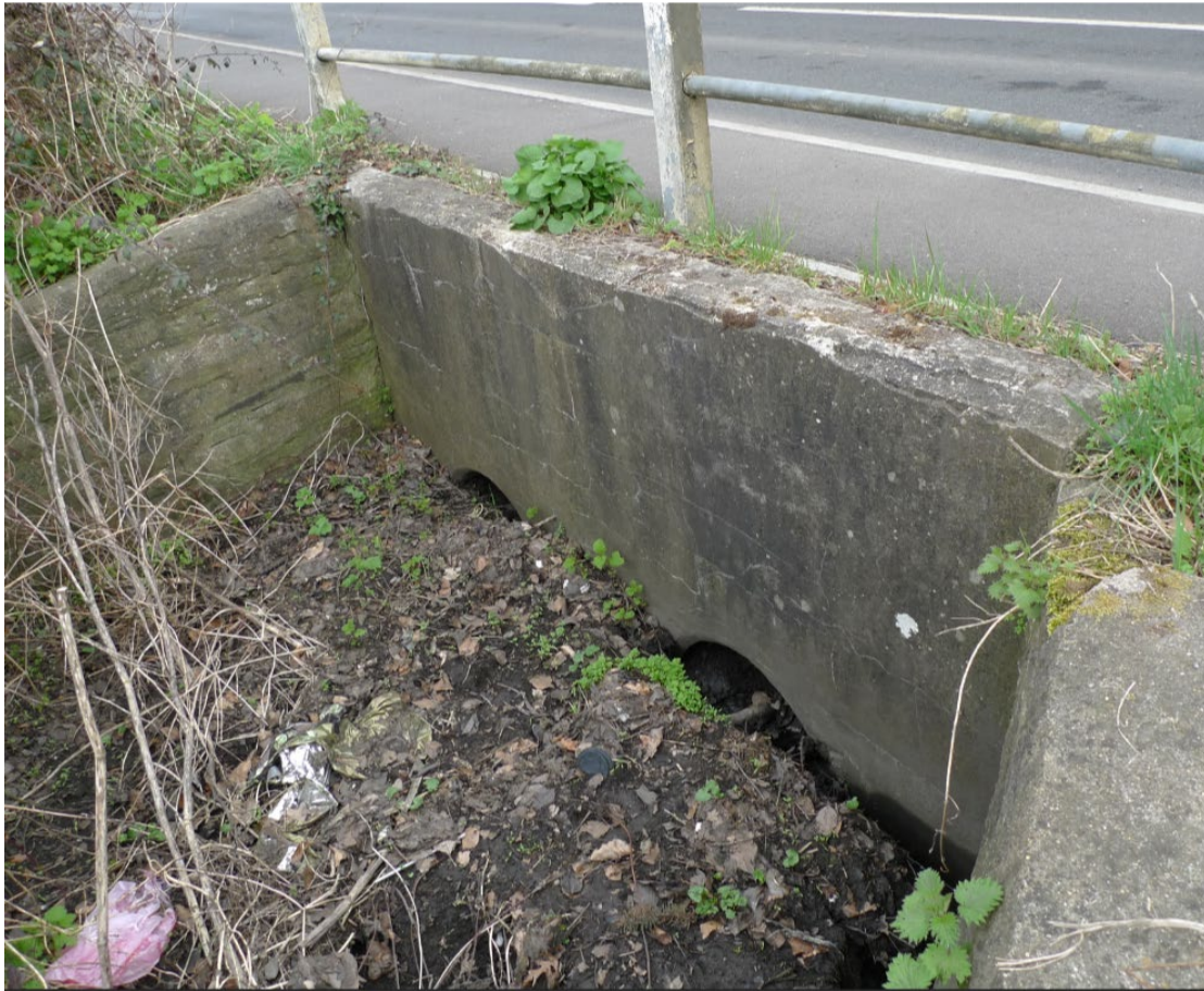
3. Upstream side of culvert under A4155.
