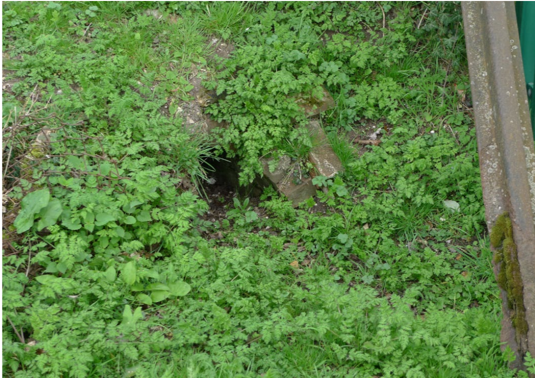
11. Outlet from very old 450mm culvert serving AFC ditch near railway culvert inlet.
