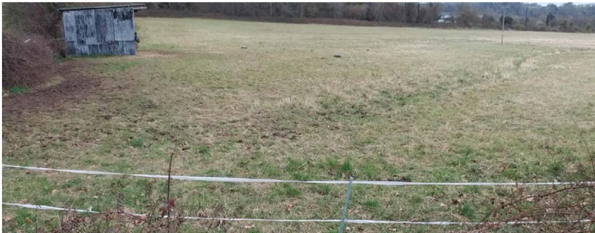
29. Route of flow (shallow channel) across horse field down to A4155 culvert.
