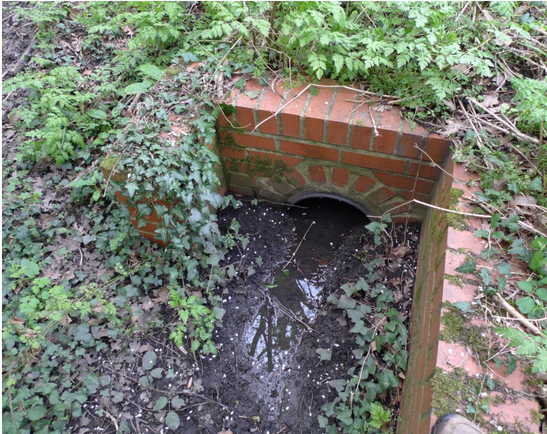
1. 375mm Culvert serving A4155 4 gullies at road low point. (Guessed).
