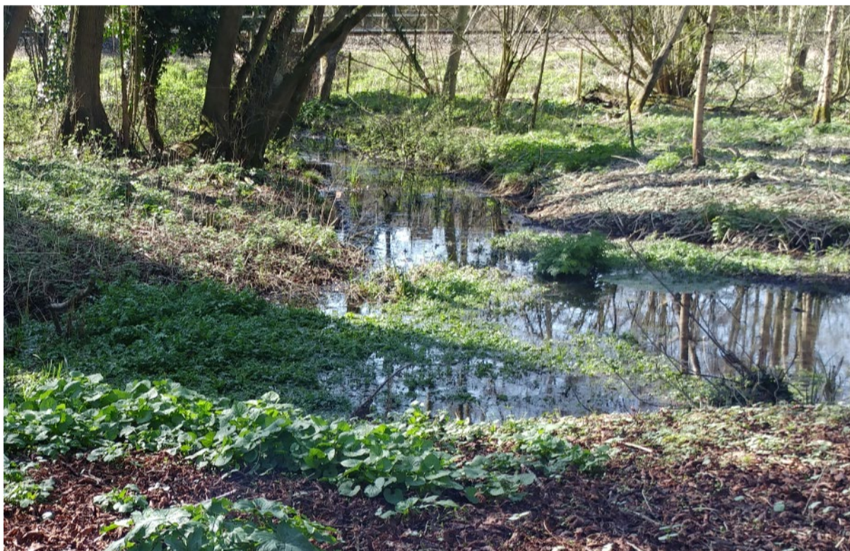
16. Main stream junction with large culvert under railway below Black Bears polo club
