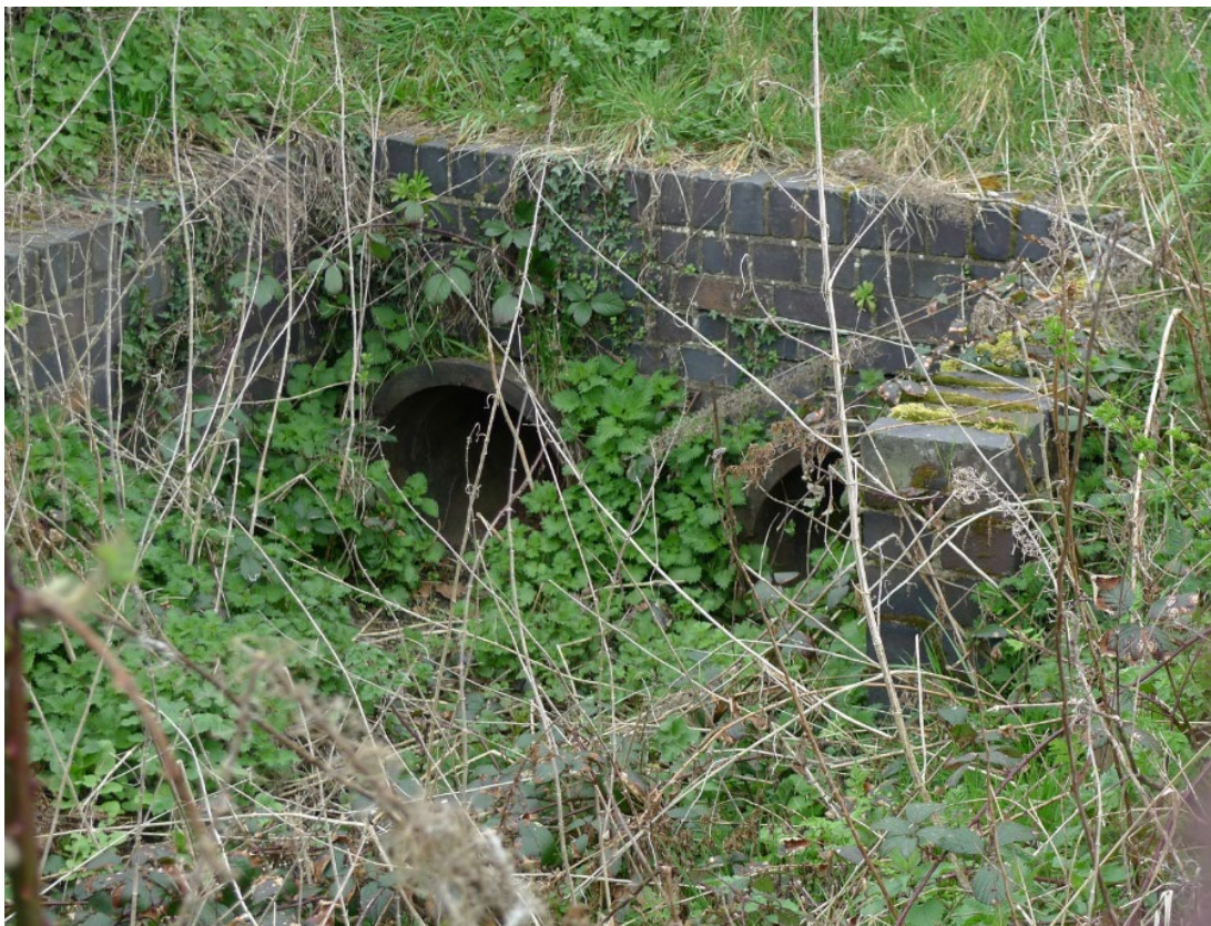
12. Railway culvert inlets. Twin 450mm?
