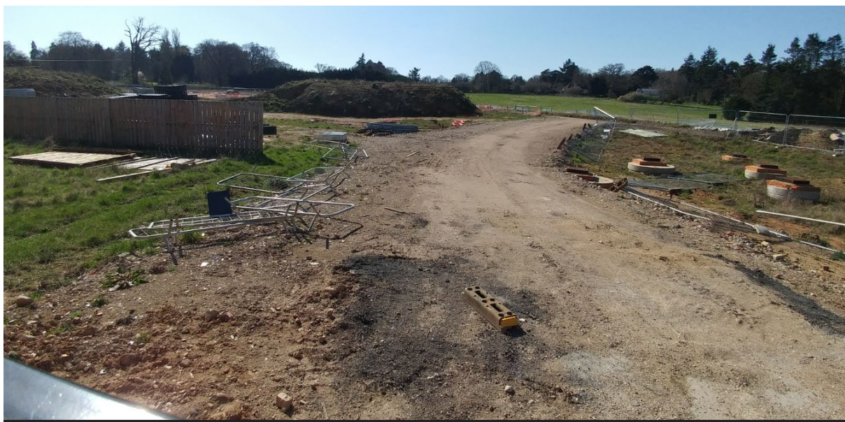
35. Site workings at Thames Farm (steep site).
