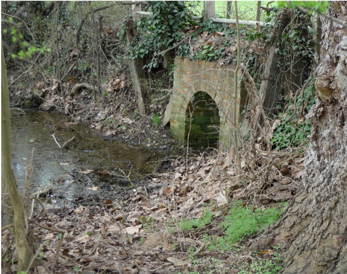
28. Culvert under road (upstream side).
