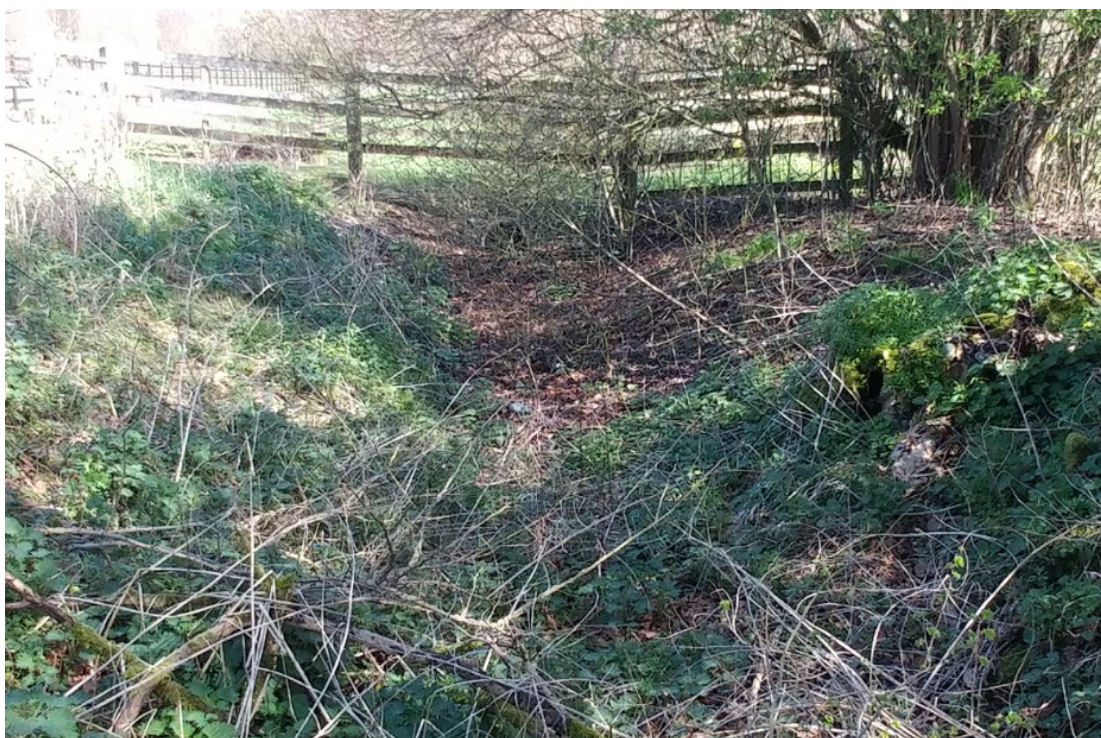
14. Looking downstream to (small) pipe from railway culvert outlet. Single 450mm / 525mm?
