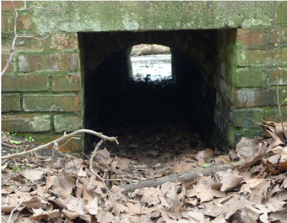
26. Culvert under road (downstream side).
