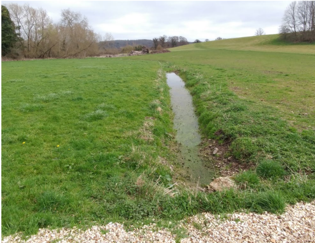
32. Downstream outlet from pond 2 x 300mm pipes). Water in channel reflecting water level in pond?
