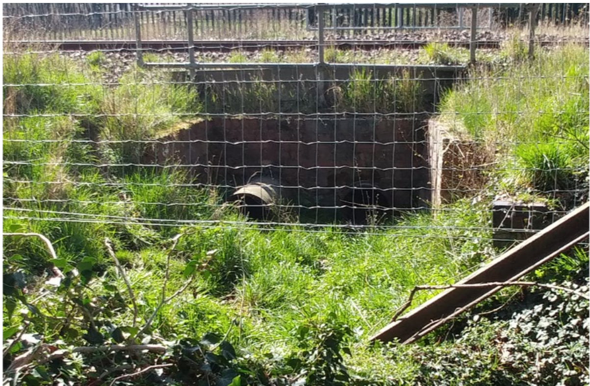
13. Railway culvert downstream outlet (smaller capacity than culvert under A4155).
