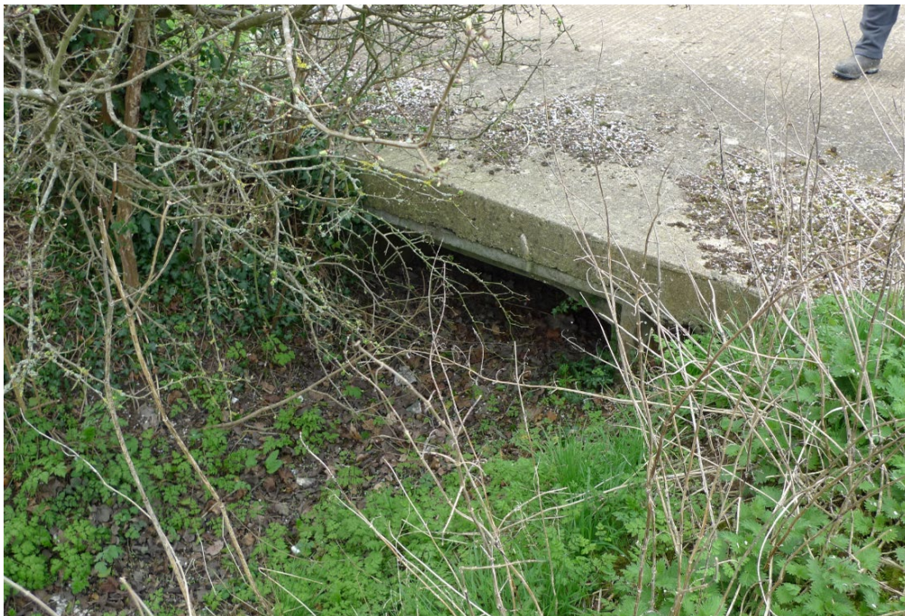
8. Box culvert half way along between A4155 and railway line in the AFC grounds
