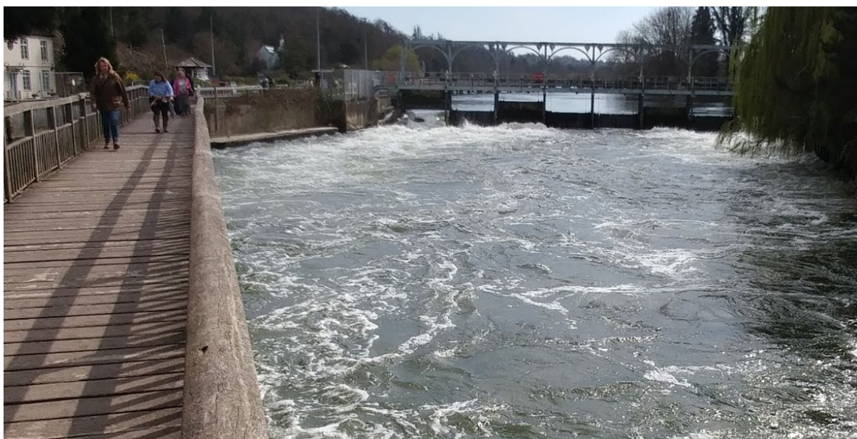
23. Water level weir control immediately upstream of outfall.
