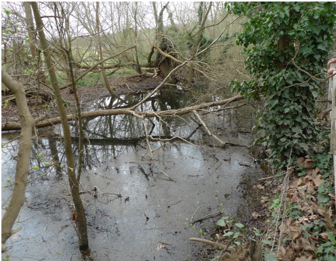
27. Ponding on upstream side of road.
