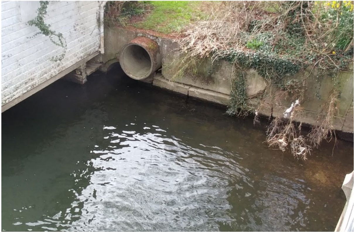
21. Outlets into R. Thames – one low level pipe, one overflow level pipe.
