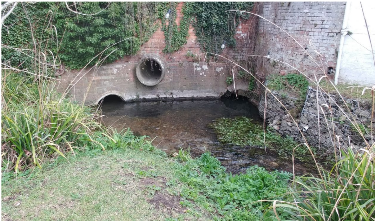
20. Outfall to River Thames by Mill Lane.
