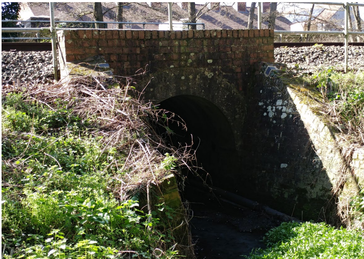
17. Railway culvert from Black Bears Polo club
