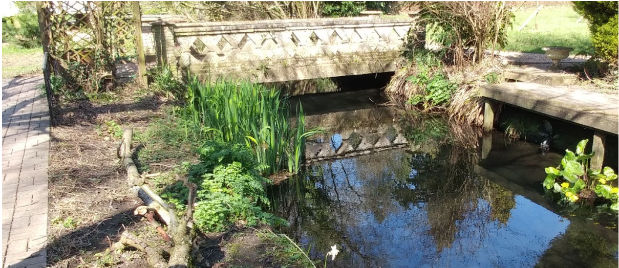
24. Many small bridges across stream along Mill Lane
