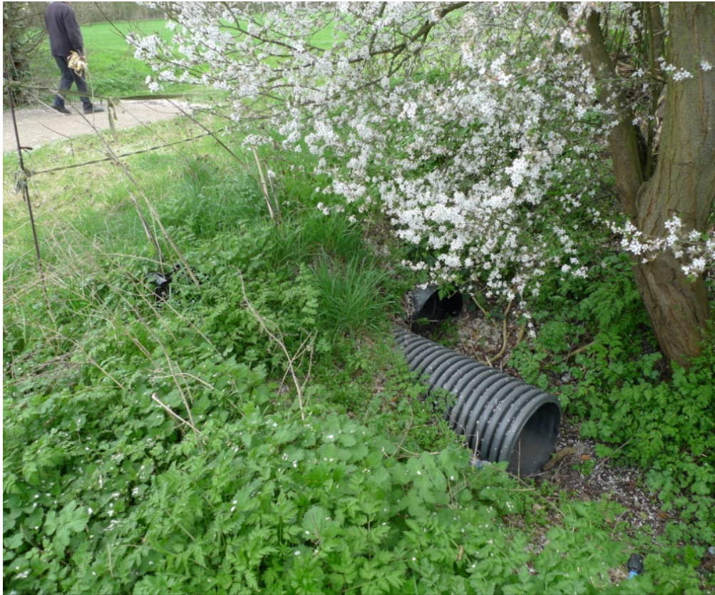
7. pipes entering box culvert half way along between A4155 and railway line in the AFC grounds
