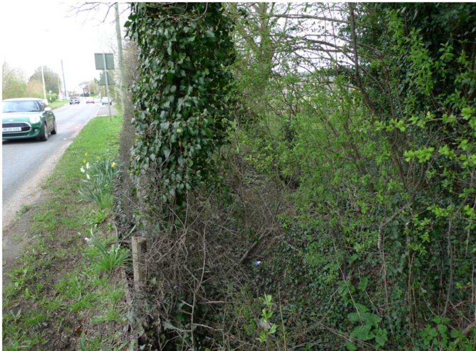
6. Looking north from culvert exit with ditch connecting to ditch 5m away beside AFC grounds.
